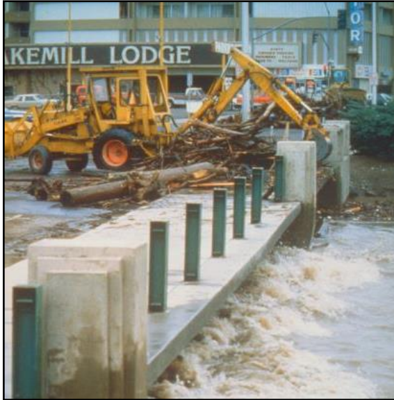
Lake Street Bridge Debris Removal
