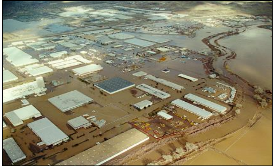
Sparks Industrial Area
